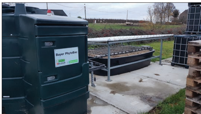
Phytobac system at the Bayer Forward Farm for pesticide residue remediation for sprayer wash water.
