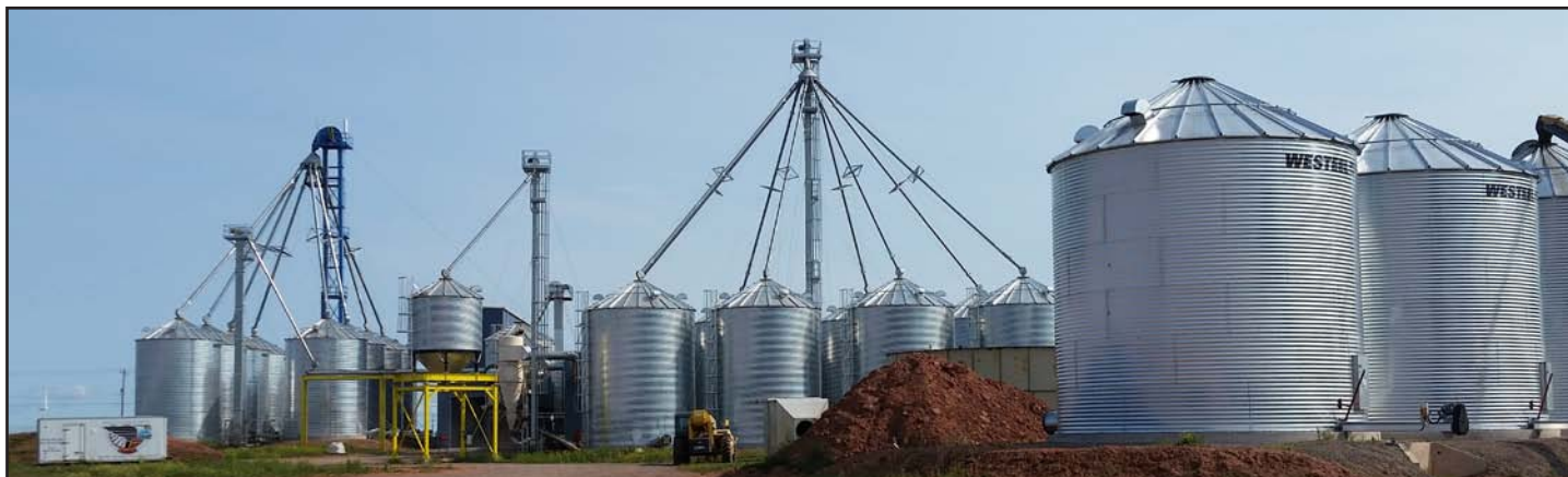
W.A. Grain & Pulse Solutions were busy early in 2018 getting storage and cleaning facilities ready in Slemon Park for harvest season. The storage tanks are in three groups - left: tanks to receive raw product from the fields; center: storage tanks for cleaned peas; right : seed storage tanks. Photo: M.K. Sonier
