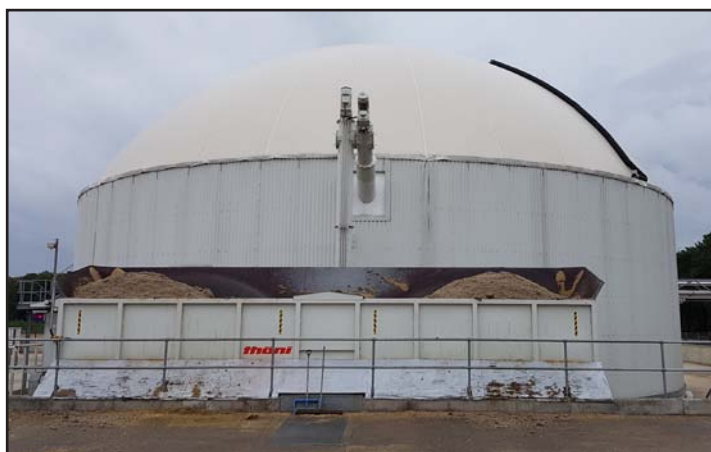
Above: Anaerobic digester at the Abrey Farm.
