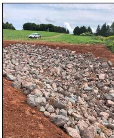
A rock chute with R25 granite rock
