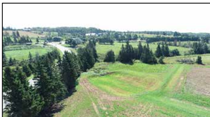
An excellent example of a sediment pond at the outlet of a soil conservation project.
